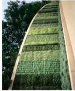
Vertical Green Wall
